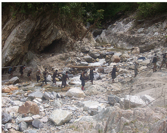
Transporting Conductor for 132kV-Gyelpozhing-Nangkhor line
