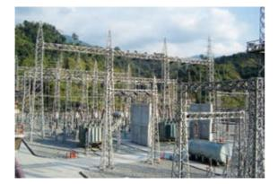
supply arrangement for Pasakha Industrial Estate, covering 3 x 63 MVA, 220/66 kV Malbase Substation, 66 kV quadruple circuit from Malbase to Pasakha, 66 kV terminal gantry and 66 kV underground distribution at Pasakha. The substation was formerly inaugurated on November 9, 2008 by Lyonpo Khandu Wangchuk, Ministry of Economic Affairs.
