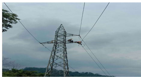
Construction of 33 kV special towers from Nuini to Talabasti
