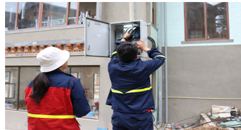
Configuration of Customer Premises Equipment for communication.
