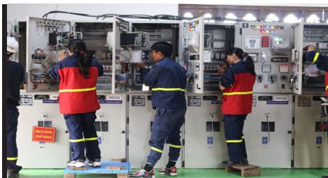
Master tripping relay installation
