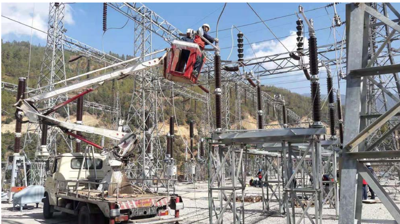
Retrofitting of Isolator at 220kV Semtokha substation
