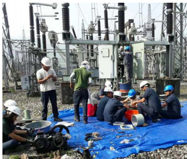
Breaker overhauling at 400kV Malbase substation
