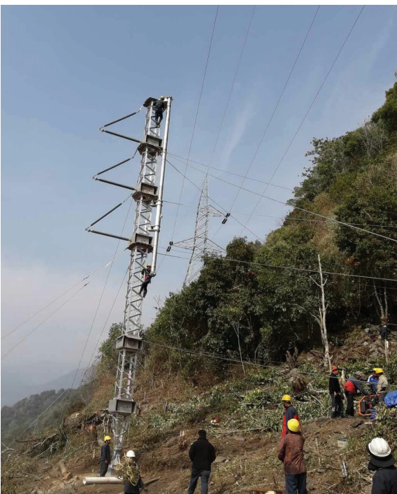
>> Figure 2: Emergency Restoration of TY55 (132kV Tintibi-Yurmoo transmission line)
