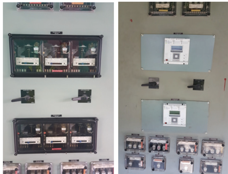
>> Figure 3. : Retrofitting of MiCOM P14 relays
