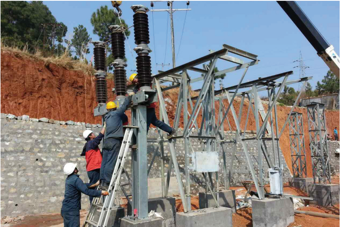
>> Figure 1: Bay Extension at Lobeyssa Substation.
